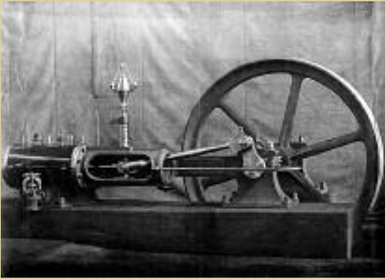
Die 1888 in Betrieb genommene Dampfmaschine The Steam-Engine taken into Operation in 1888
